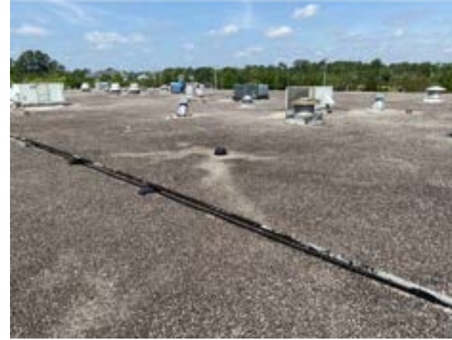
PHOTO # 4 ROOF AREA B
