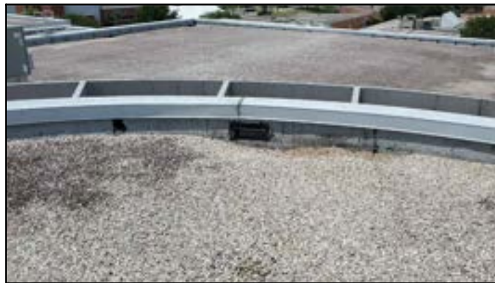
PHOTO # 8 ROOF AREA A1
