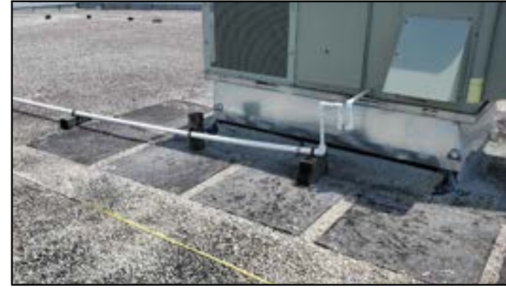
PHOTO # 27 ROOF AREA C
