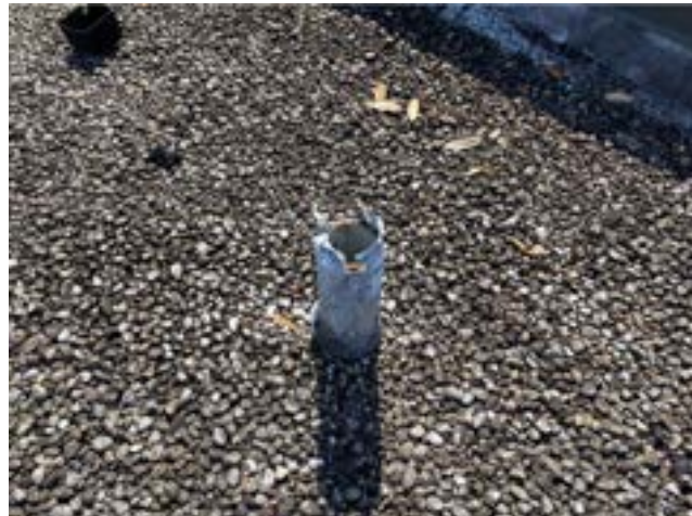
PHOTO # 11 ROOF AREA D
