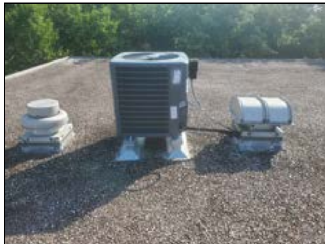
PHOTO # 10 ROOF AREA A
