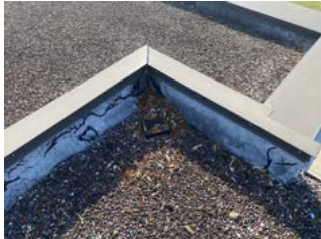
PHOTO # 6 ROOF AREA F
