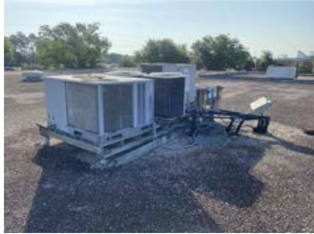
PHOTO # 3 ROOF AREA F
