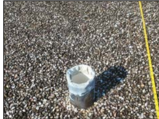
PHOTO # 8 ROOF AREA A
