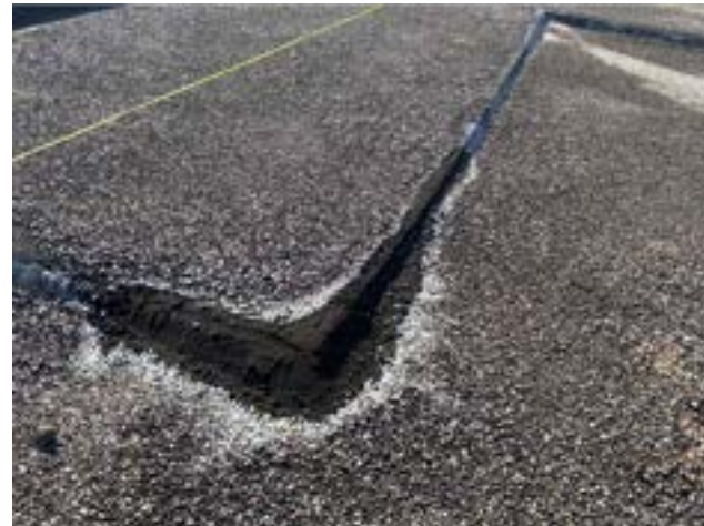
PHOTO # 11 ROOF AREA C i
