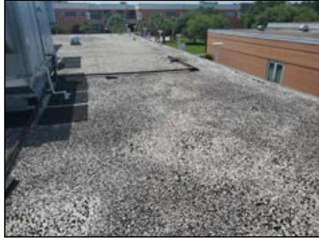
PHOTO # 1 ROOF AREA A
