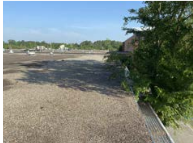
PHOTO # 5 ROOF AREA F
