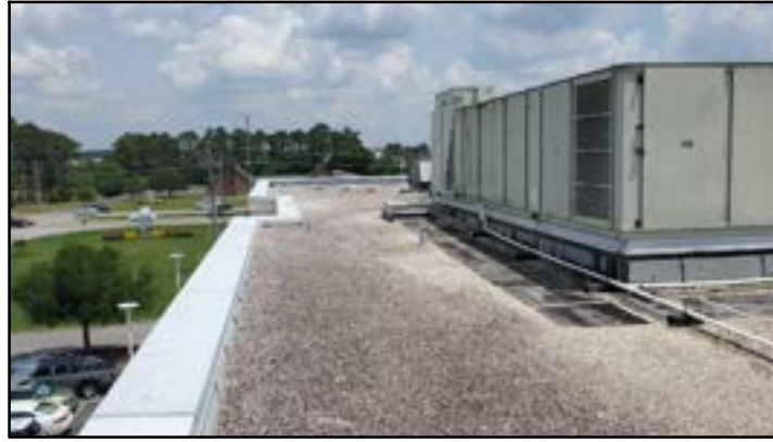
PHOTO # 14 ROOF AREA B
