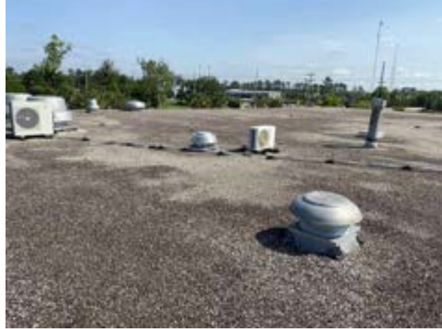
PHOTO # 7 ROOF AREA D
