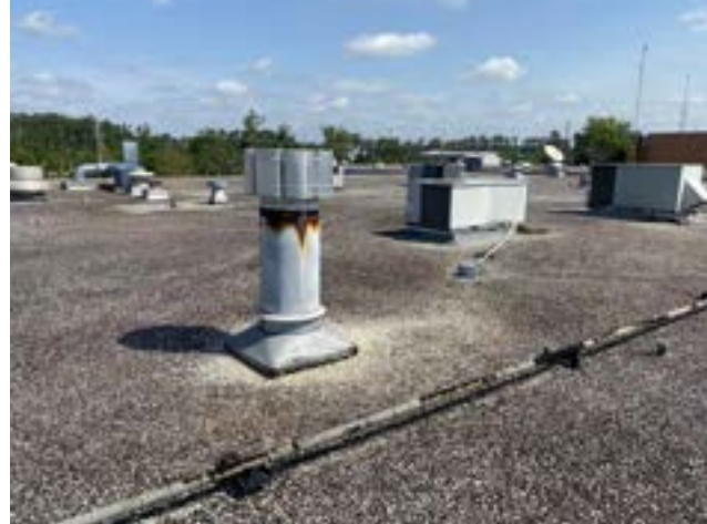
PHOTO # 5 ROOF AREA B
