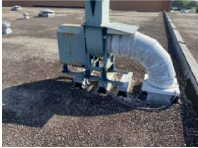
PHOTO # 2 ROOF AREA E
