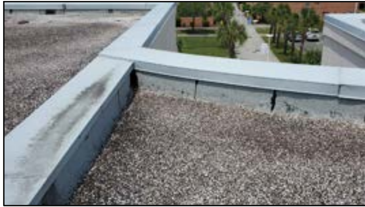
PHOTO # 28 ROOF AREA C
