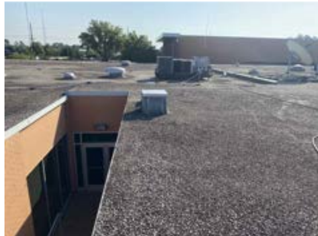
PHOTO # 9 ROOF AREA C
