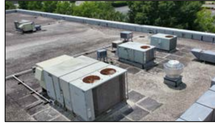
PHOTO # 39 ROOF AREA E
