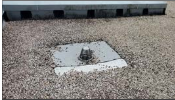
PHOTO # 17 ROOF AREA B
