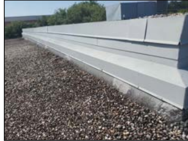
PHOTO # 4 ROOF AREA A
