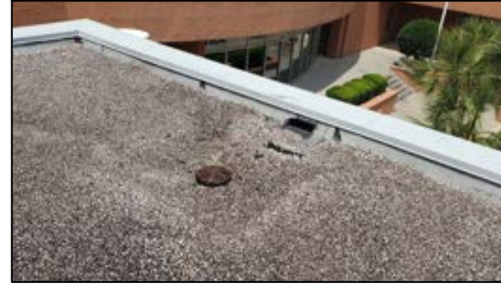
PHOTO # 48 ROOF AREA G
