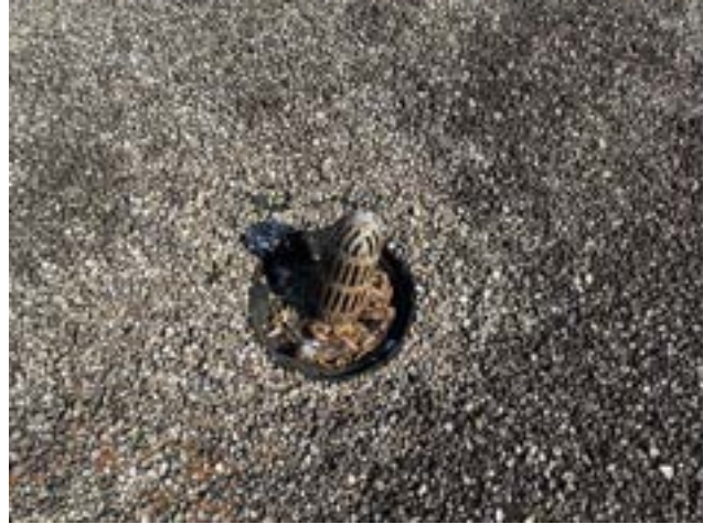
PHOTO # 8 ROOF AREA E
