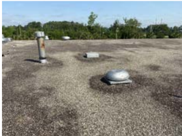
PHOTO # 10 ROOF AREA D
