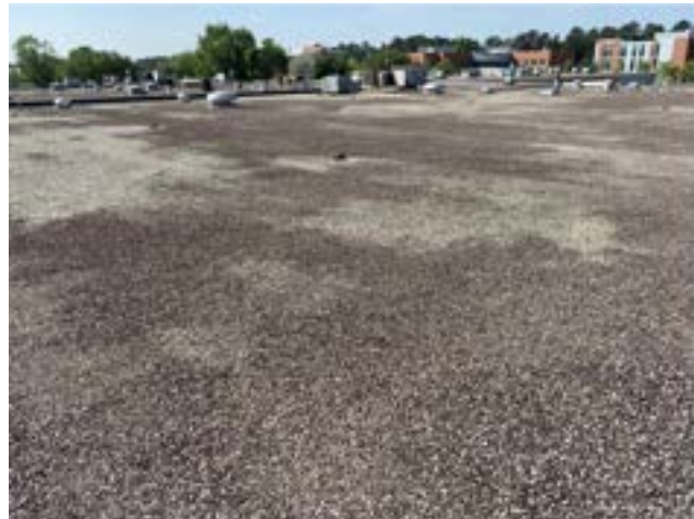
PHOTO # 12 ROOF AREA D
