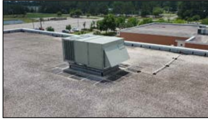
PHOTO # 2 ROOF AREA A
