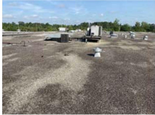
PHOTO # 1 ROOF AREA E
