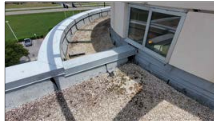
PHOTO # 9 ROOF AREA A2
