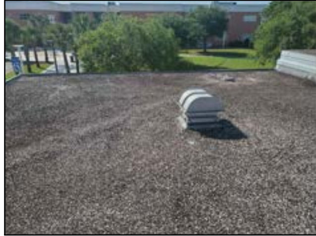
PHOTO # 1 ROOF AREA A
