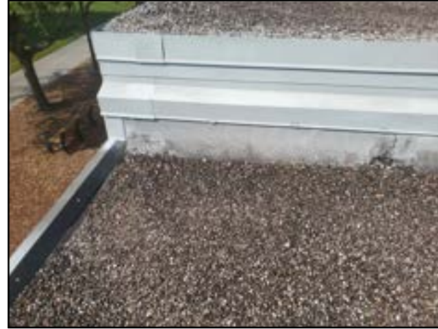
PHOTO # 3 ROOF AREA A
