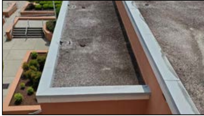
PHOTO # 47 ROOF AREA G
