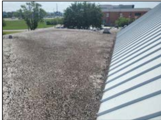
PHOTO # 11 ROOF AREA B
