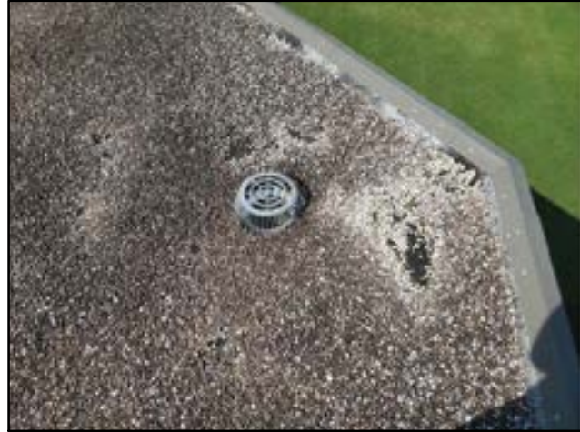
PHOTO # 5 ROOF AREA A
