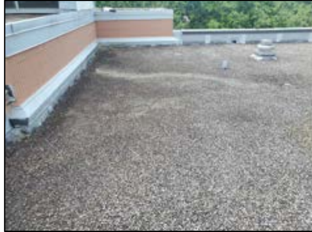
PHOTO # 5 ROOF AREA A
