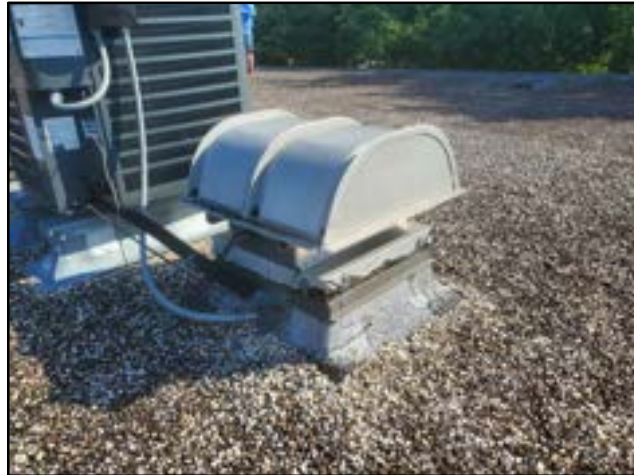
PHOTO # 6 ROOF AREA A
