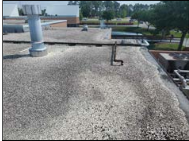
PHOTO # 5 ROOF AREA A
