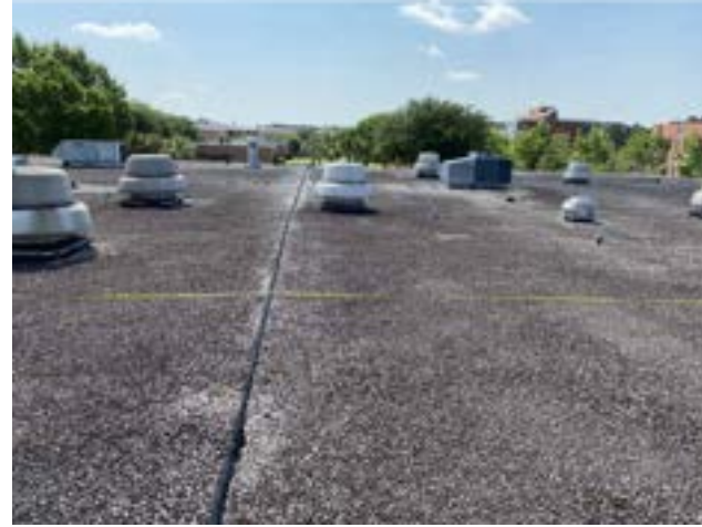
PHOTO # 3 ROOF AREA A
