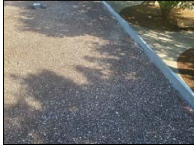
PHOTO # 3 ROOF AREA A
