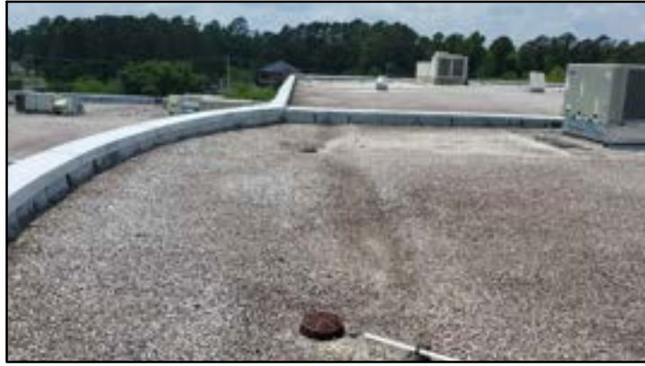
PHOTO # 25 ROOF AREA C
