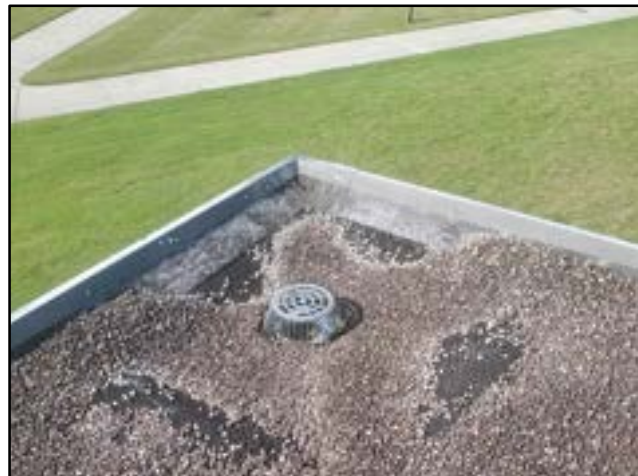
PHOTO # 9 ROOF AREA A
