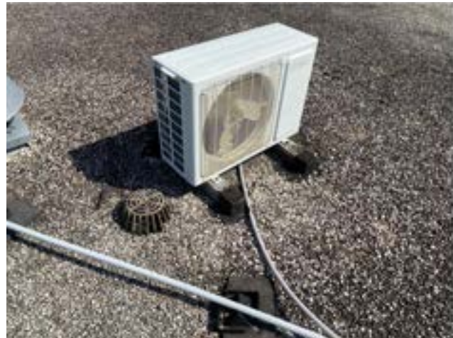
PHOTO # 9 ROOF AREA D
