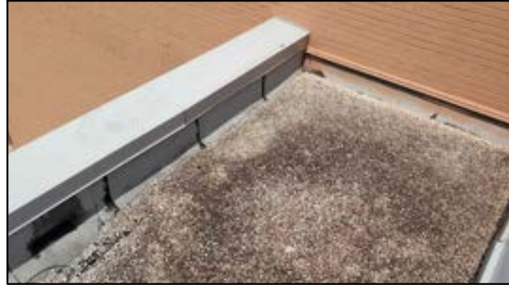
PHOTO # 46 ROOF AREA F
