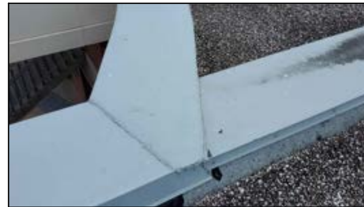
PHOTO # 33 ROOF AREA D
