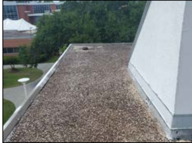
PHOTO # 7 ROOF AREA B
