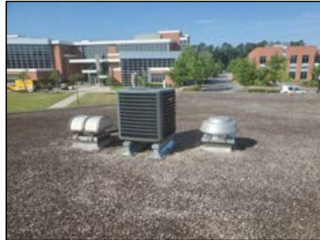
PHOTO # 7 ROOF AREA A
