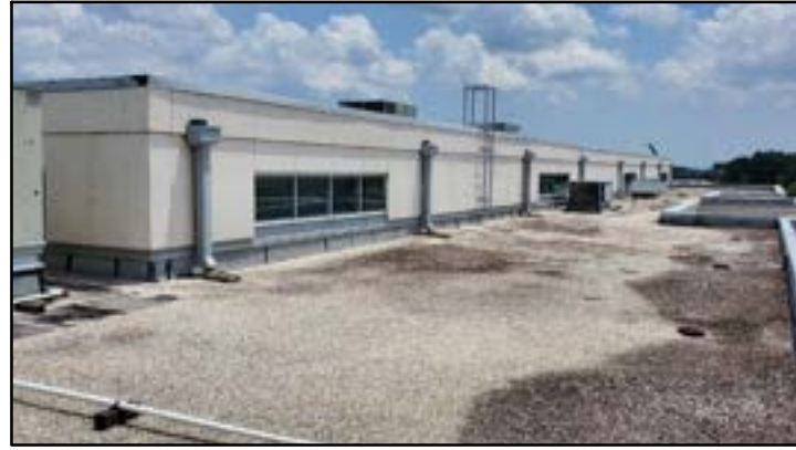
PHOTO # 13 ROOF AREA B
