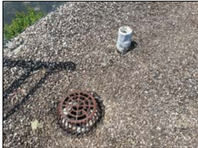
PHOTO # 11 ROOF AREA C
