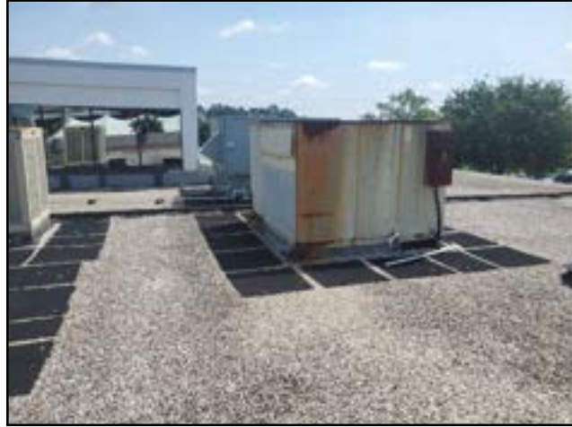
PHOTO # 4 ROOF AREA A
