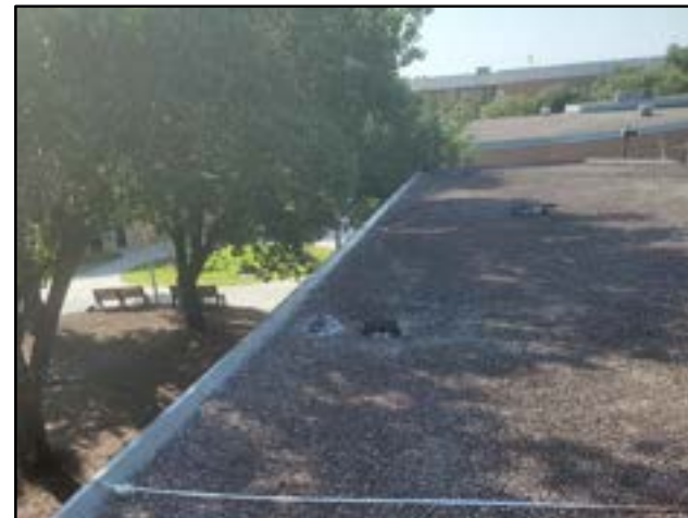
PHOTO # 12 ROOF AREA A
