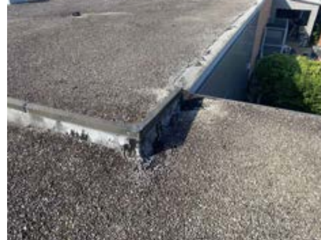
PHOTO # 8 ROOF AREA C
