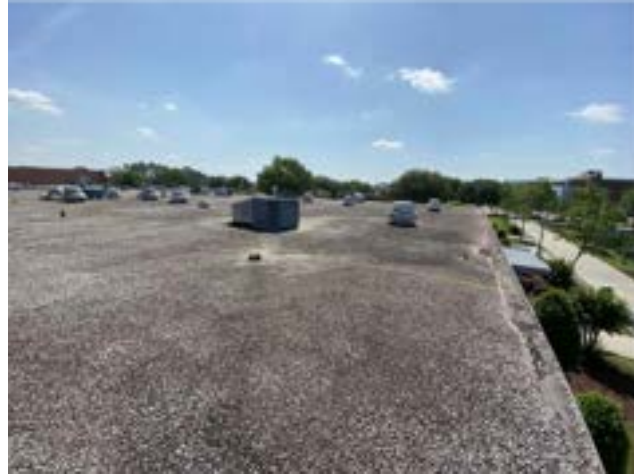
PHOTO # 2 ROOF AREA A
