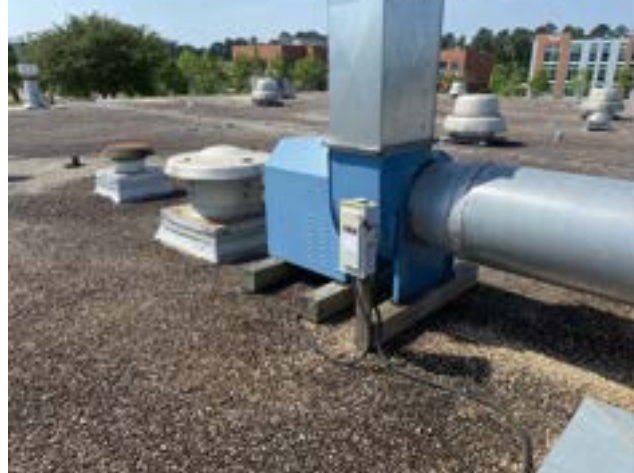
PHOTO # 6 ROOF AREA B
