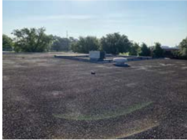
PHOTO # 2 ROOF AREA F
