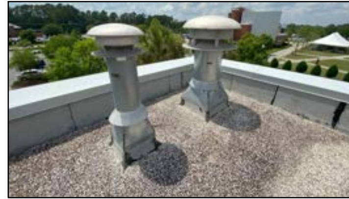
PHOTO # 42 ROOF AREA E
