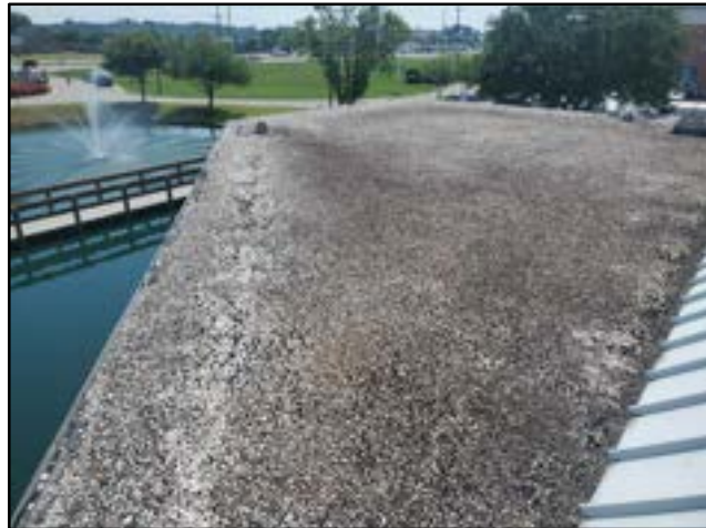
PHOTO # 10 ROOF AREA B
