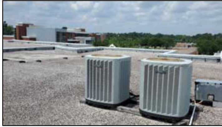
PHOTO # 26 ROOF AREA C
