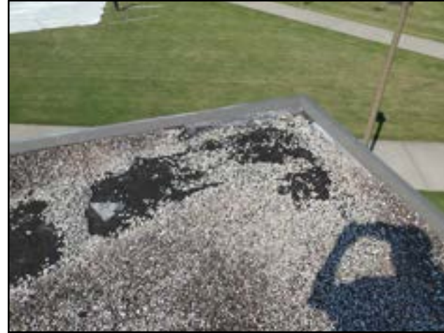
PHOTO # 7 ROOF AREA A
