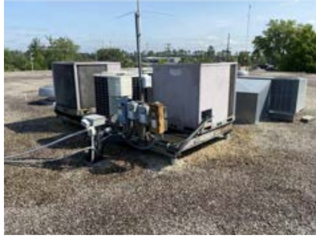
PHOTO # 4 ROOF AREA D
