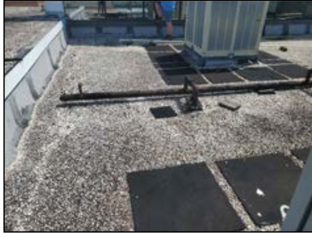
PHOTO # 2 ROOF AREA A
