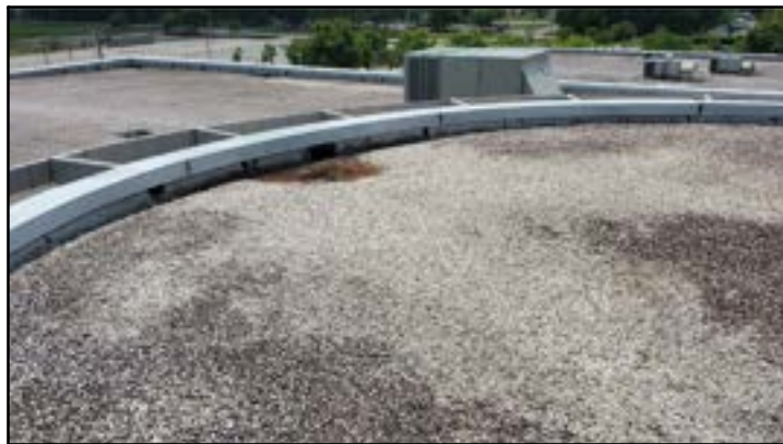
PHOTO # 7 ROOF AREA A1
