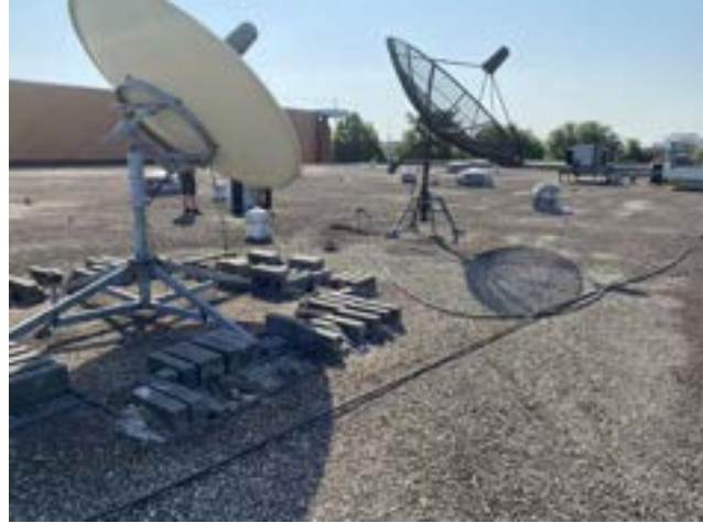
PHOTO # 7 ROOF AREA E
