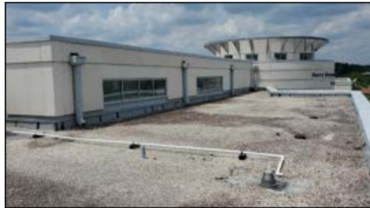
PHOTO # 22 ROOF AREA B
