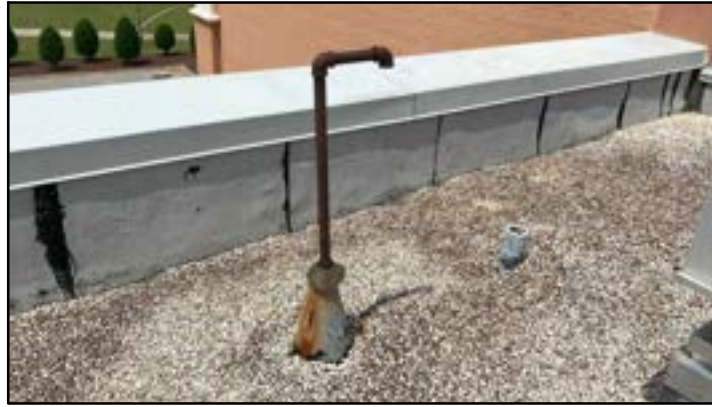
PHOTO # 44 ROOF AREA E
