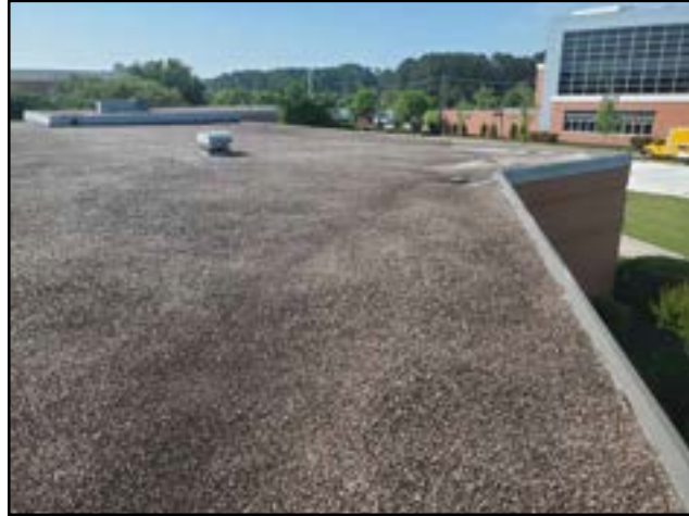
PHOTO # 6 ROOF AREA A
