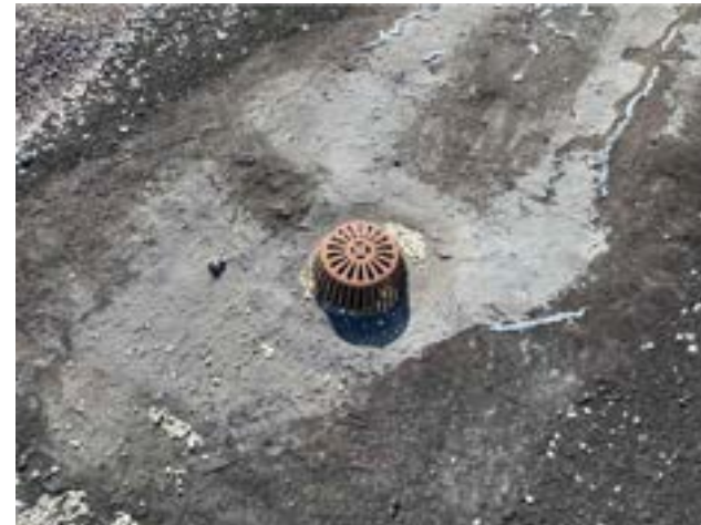
PHOTO # 12 ROOF AREA C i
