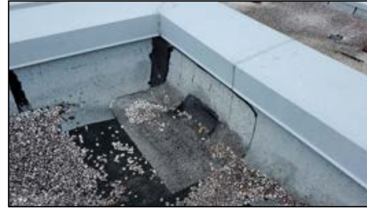
PHOTO # 3 ROOF AREA A
