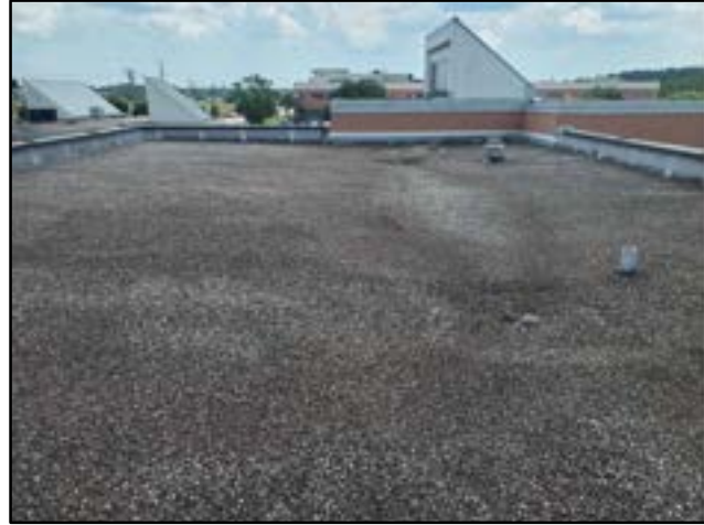
PHOTO # 1 ROOF AREA A
