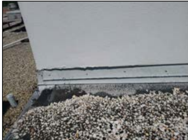
PHOTO # 12 ROOF AREA B
