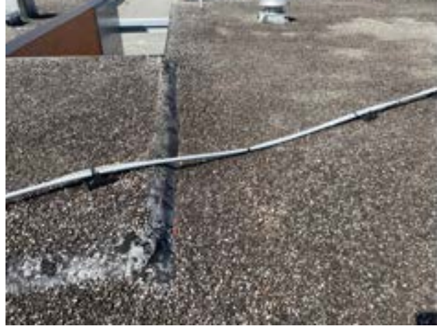
PHOTO # 8 ROOF AREA D
