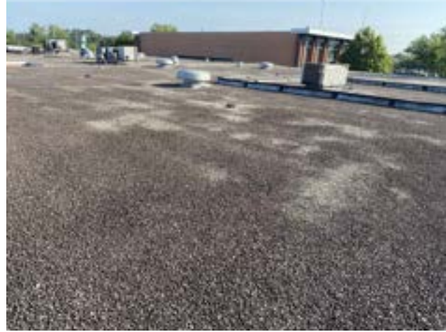
PHOTO # 1 ROOF AREA F
