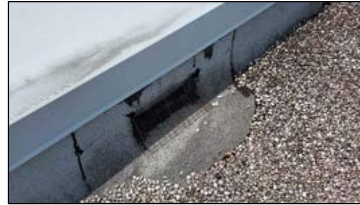
PHOTO # 30 ROOF AREA C
