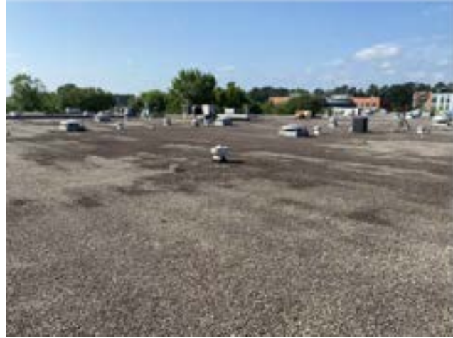
PHOTO # 4 ROOF AREA E
