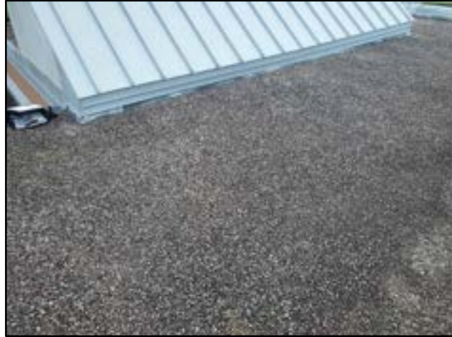
PHOTO # 8 ROOF AREA B
