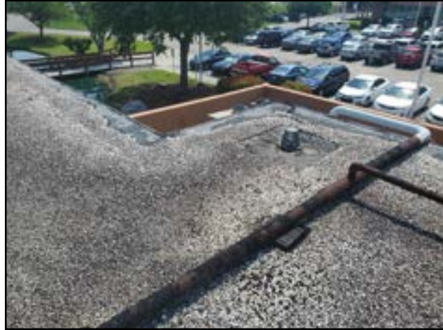
PHOTO # 6 ROOF AREA A
