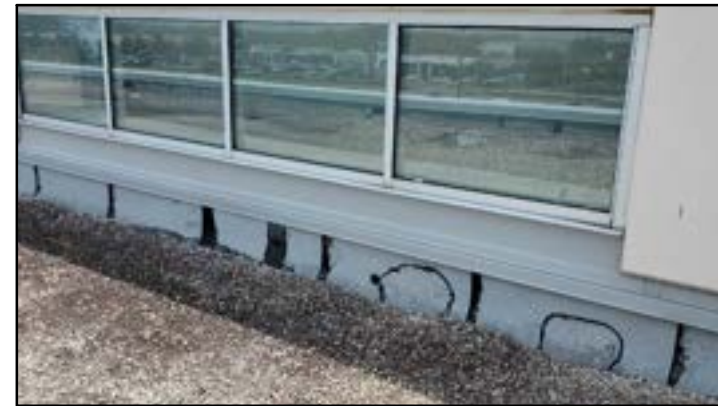
PHOTO # 24 ROOF AREA B
