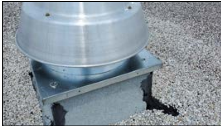
PHOTO # 35 ROOF AREA D
