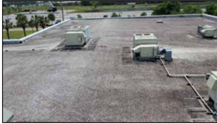
PHOTO # 38 ROOF AREA E
