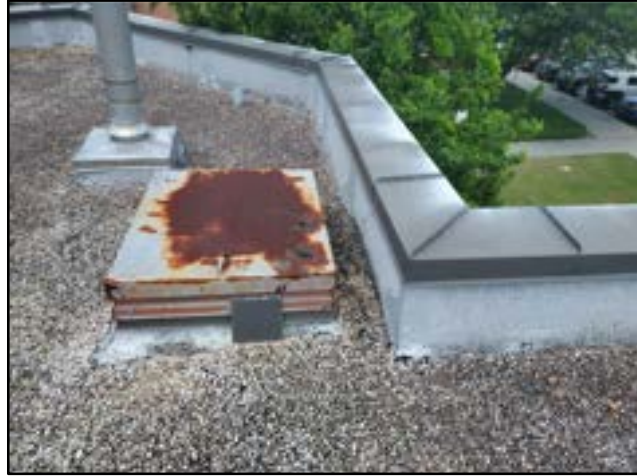
PHOTO # 2 ROOF AREA A
