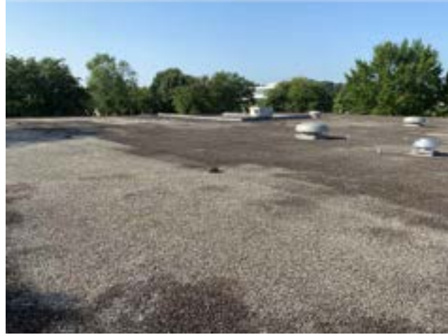
PHOTO # 4 ROOF AREA F
