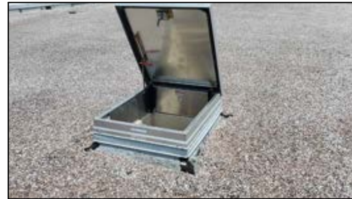
PHOTO # 36 ROOF AREA D
