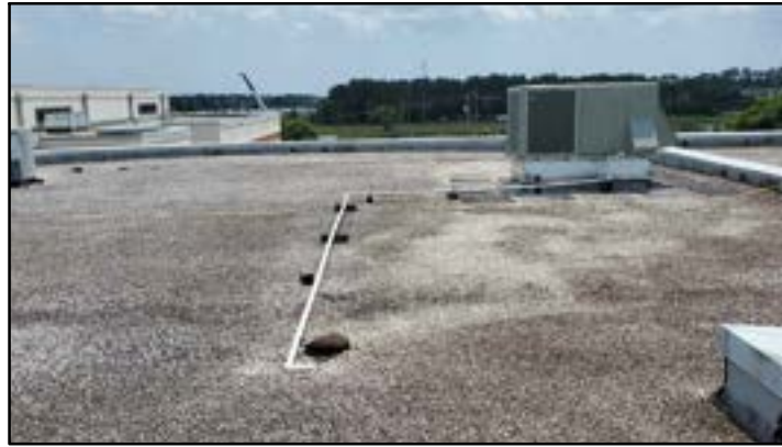
PHOTO # 29 ROOF AREA C
