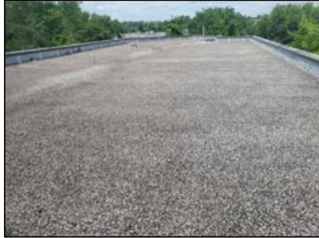
PHOTO # 3 ROOF AREA A
