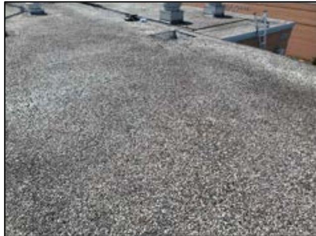
PHOTO # 9 ROOF AREA B
