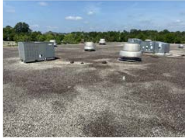
PHOTO # 1 ROOF AREA A
