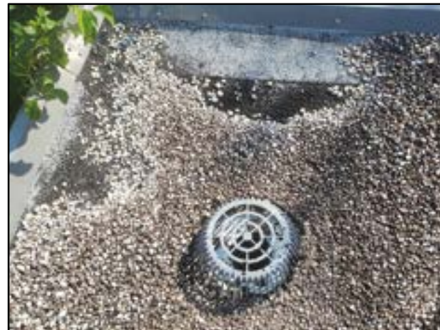
PHOTO # 11 ROOF AREA A
