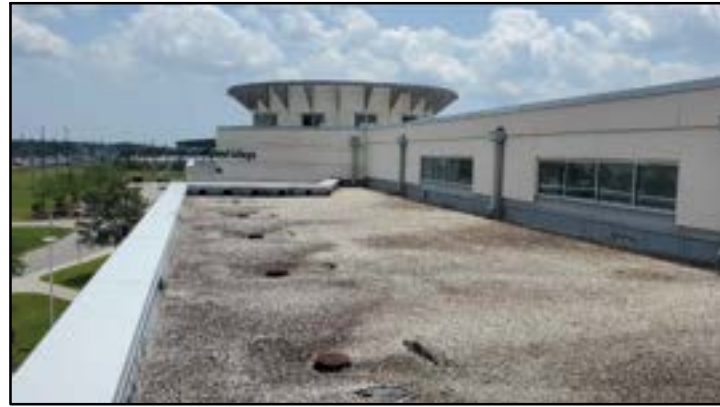
PHOTO # 16 ROOF AREA B
