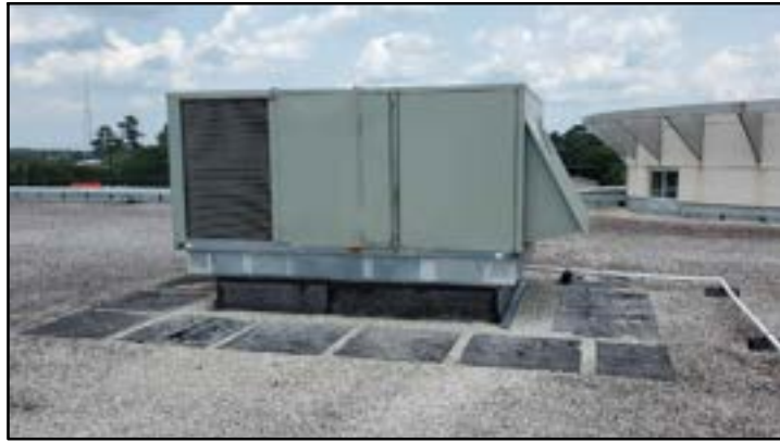
PHOTO # 4 ROOF AREA A
