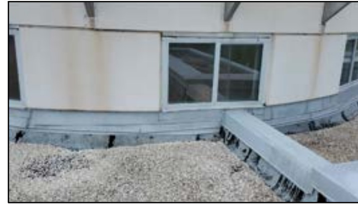
PHOTO # 6 ROOF AREA A
