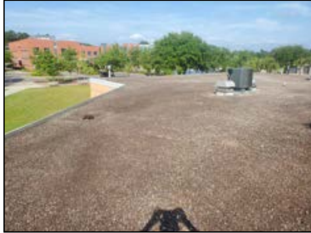
PHOTO # 2 ROOF AREA A
