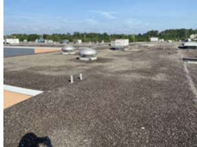
PHOTO # 7 ROOF AREA C
