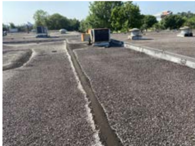
PHOTO # 10 ROOF AREA C i
