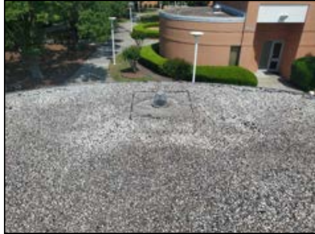
PHOTO # 7 ROOF AREA B
