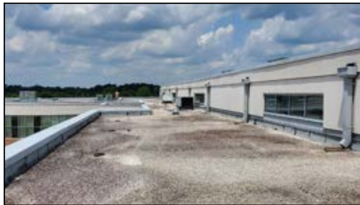
PHOTO # 20 ROOF AREA B
