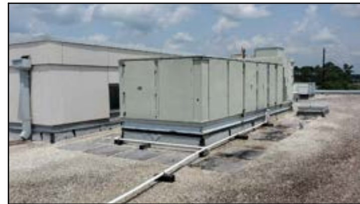
PHOTO # 21 ROOF AREA B
