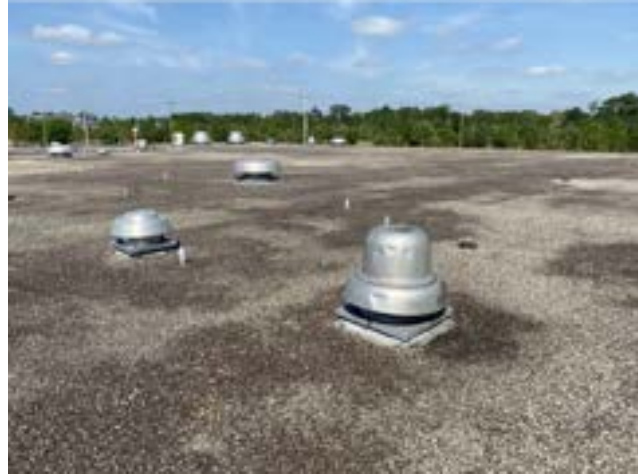
PHOTO # 3 ROOF AREA D
