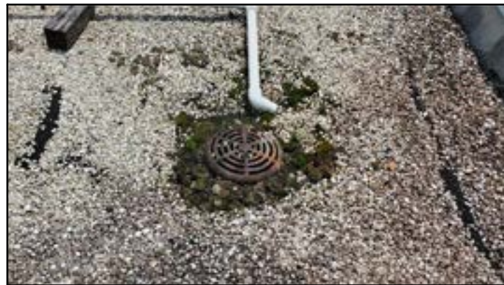
PHOTO # 19 ROOF AREA B
