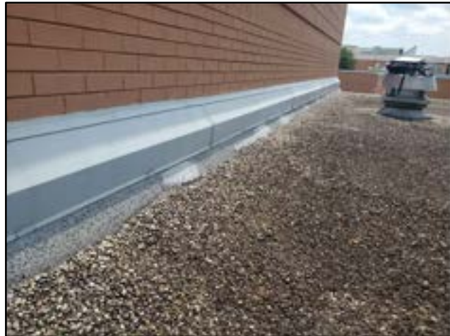
PHOTO # 12 ROOF AREA C
