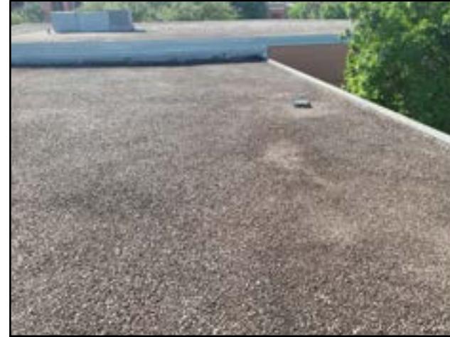
PHOTO # 8 ROOF AREA A
