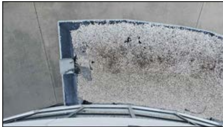
PHOTO # 11 ROOF AREA A3
