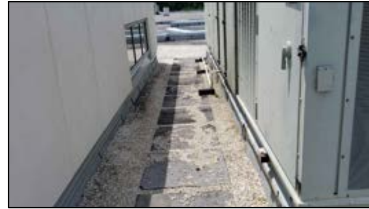
PHOTO # 18 ROOF AREA B
