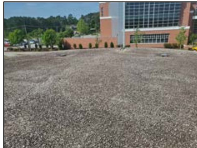
PHOTO # 11 ROOF AREA B
