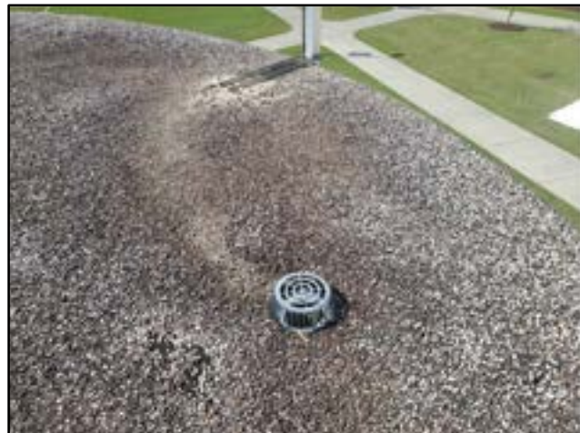
PHOTO # 9 ROOF AREA B
