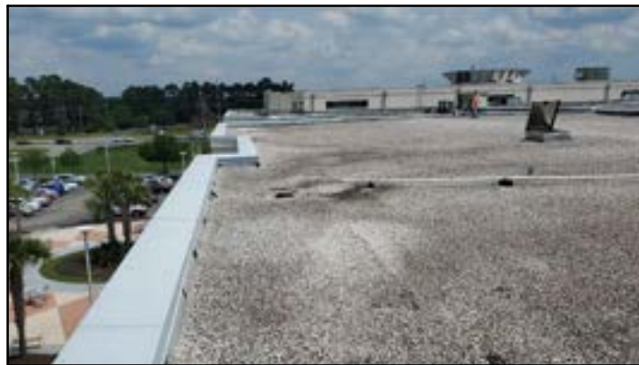
PHOTO # 32 ROOF AREA D
