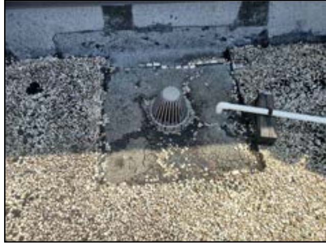
PHOTO # 3 ROOF AREA A
