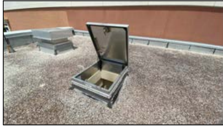
PHOTO # 43 ROOF AREA E
