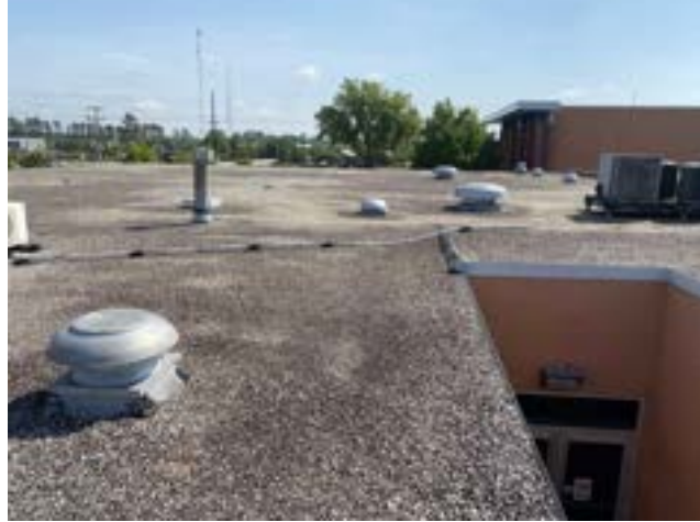
PHOTO # 6 ROOF AREA D
