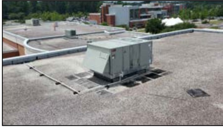
PHOTO # 1 ROOF AREA A
