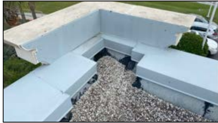
PHOTO # 40 ROOF AREA E
