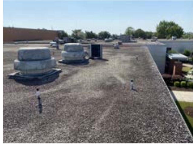
PHOTO # 1 ROOF AREA D
