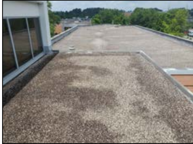
PHOTO # 6 ROOF AREA B
