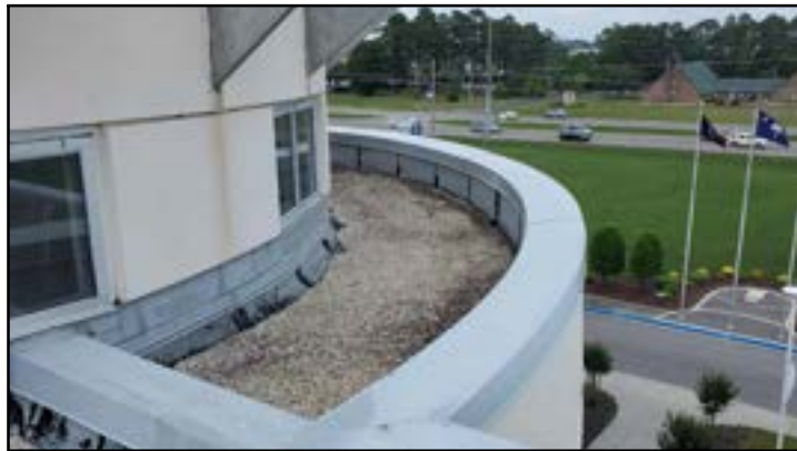
PHOTO # 10 ROOF AREA A2
