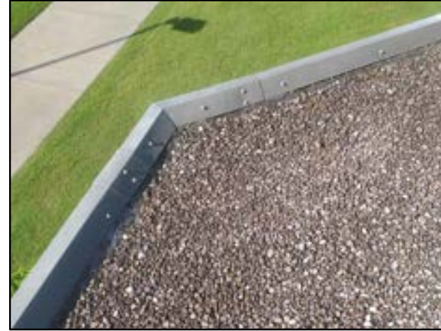
PHOTO # 4 ROOF AREA A
