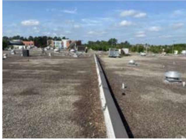
PHOTO # 3 ROOF AREA E
