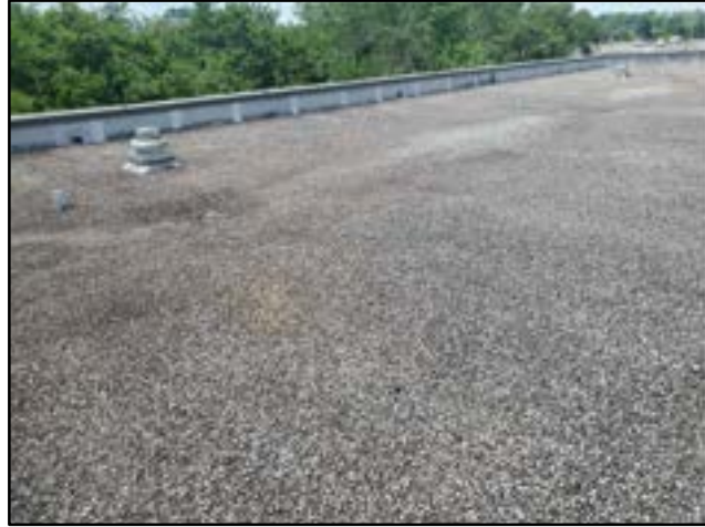
PHOTO # 4 ROOF AREA A
