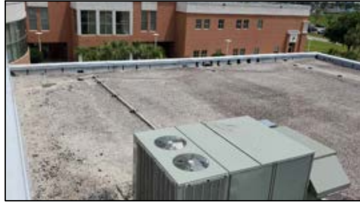
PHOTO # 37 ROOF AREA E
