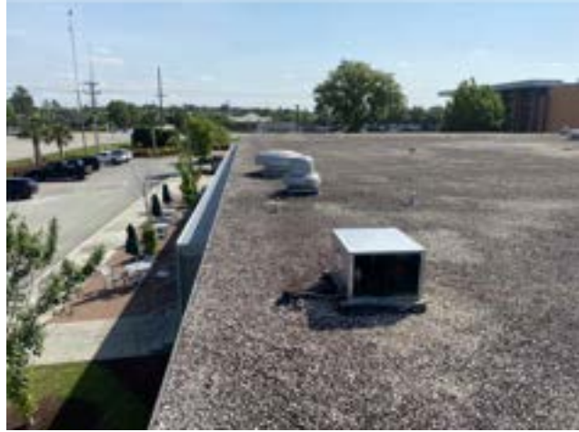
PHOTO # 2 ROOF AREA D
