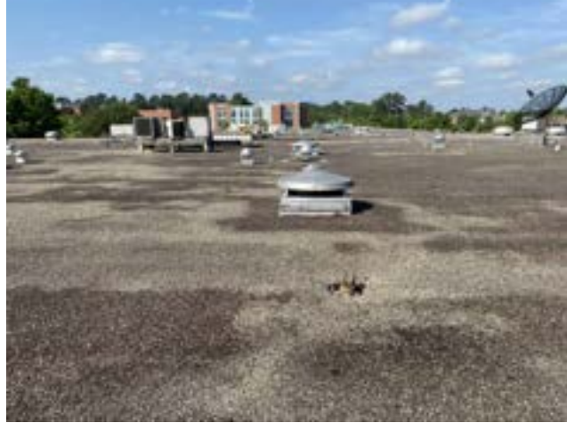
PHOTO # 6 ROOF AREA E
