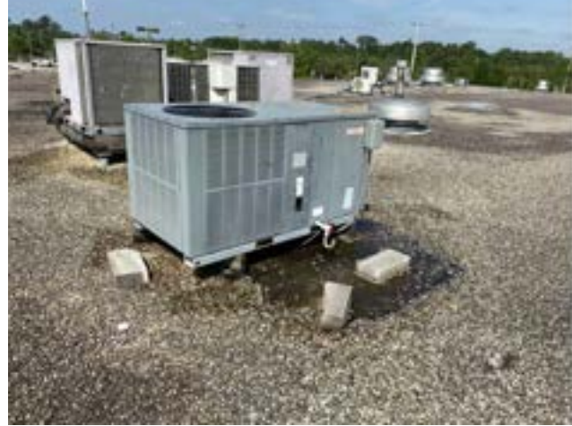
PHOTO # 5 ROOF AREA D
