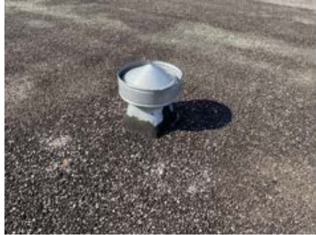
PHOTO # 5 ROOF AREA E
