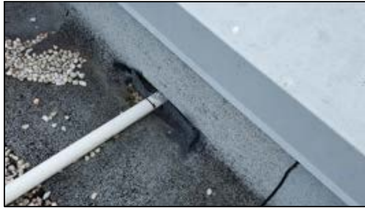
PHOTO # 5 ROOF AREA A
