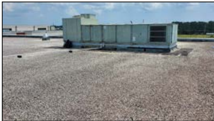
PHOTO # 31 ROOF AREA D
