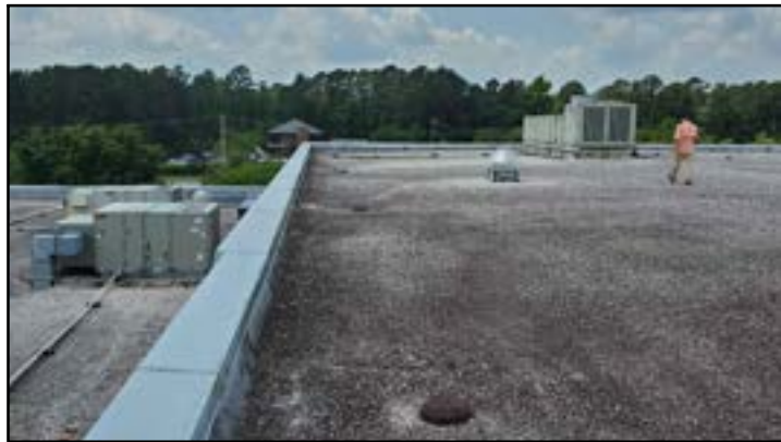
PHOTO # 34 ROOF AREA D
