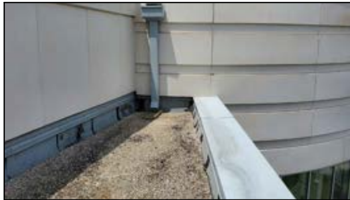
PHOTO # 23 ROOF AREA B
