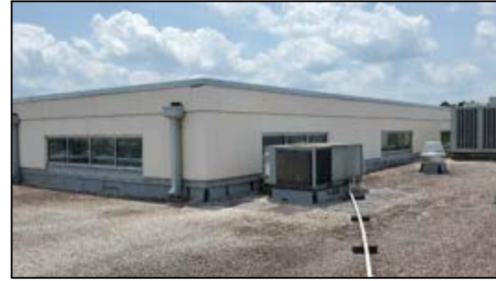
PHOTO # 15 ROOF AREA B
