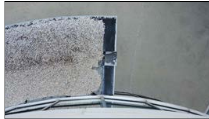
PHOTO # 12 ROOF AREA A3
