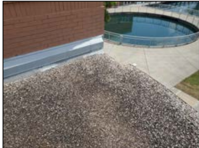
PHOTO # 9 ROOF AREA C
