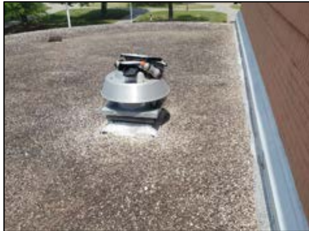
PHOTO # 10 ROOF AREA C
