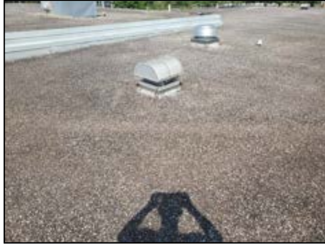
PHOTO # 2 ROOF AREA A
