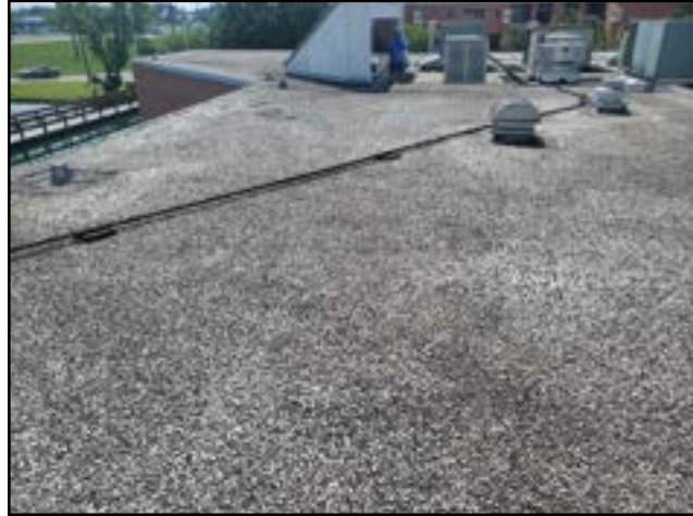
PHOTO # 8 ROOF AREA B
