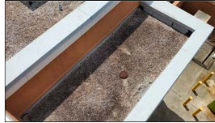
PHOTO # 45 ROOF AREA F
