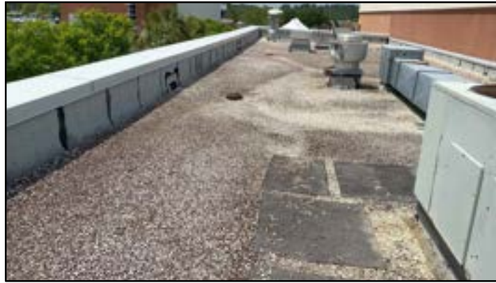
PHOTO # 41 ROOF AREA E
