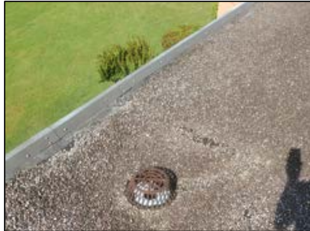
PHOTO # 5 ROOF AREA A
