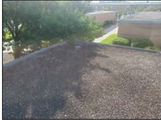
PHOTO # 1 ROOF AREA A
