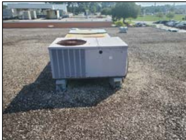
PHOTO # 10 ROOF AREA B
