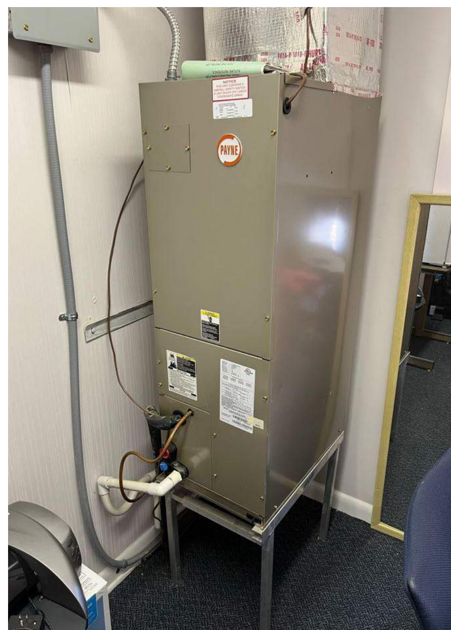
4 BUILDING 900 TYPICAL INDOOR UNIT SCALE: NTS
