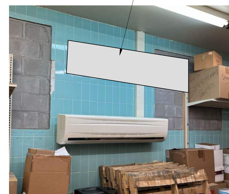
6 BUILDING 200 MINISPLIT FAN COIL-DLSS-2 M102A SCALE: NTS
