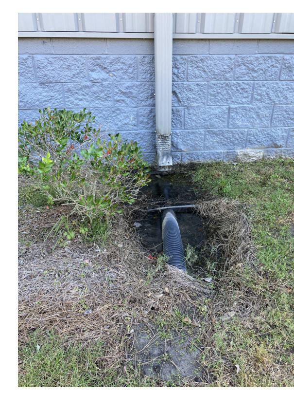
NORTH ELEVATION - EXISTING DRAIN AT DOWNSPOUT
