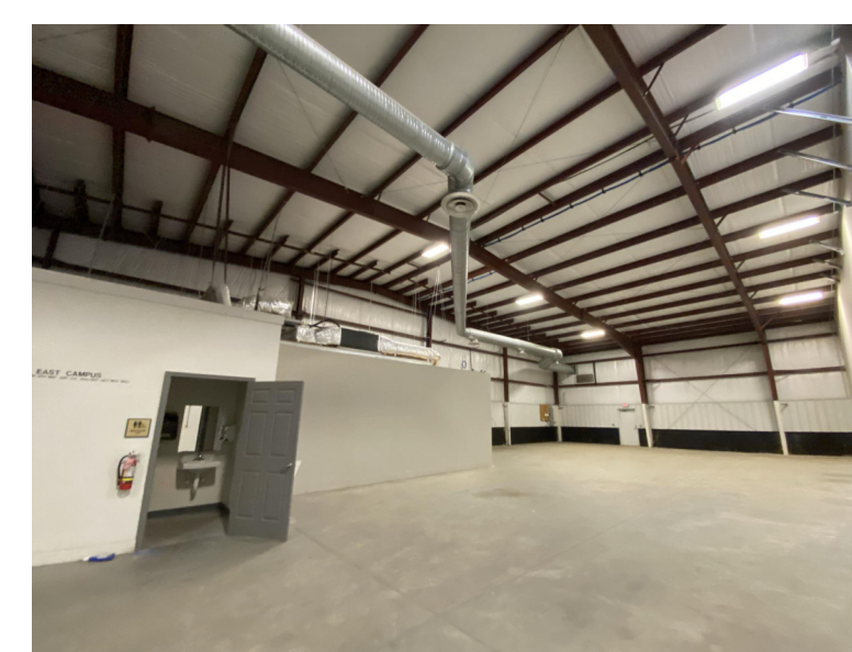
WAREHOUSE WEST SIDE - LOOKING NORTH WEST
