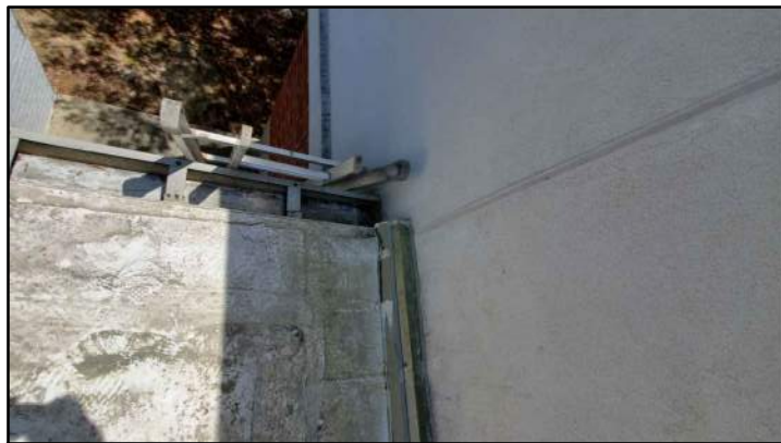
PHOTO # 7 ROOF AREA A1
