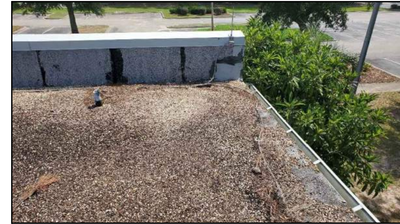
PHOTO # 3 ROOF AREA B
