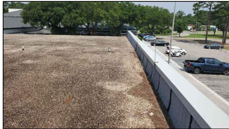
PHOTO # 4 ROOF AREA B
