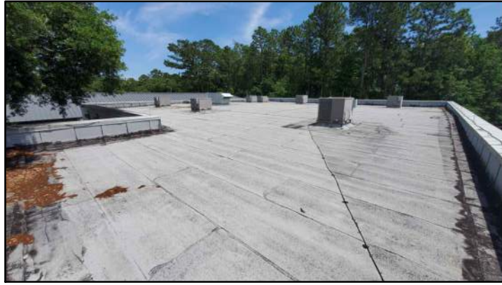
PHOTO # 1 ROOF AREA A
