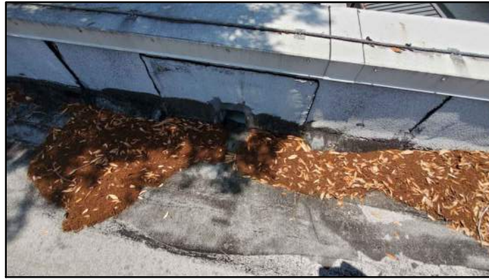
PHOTO # 5 ROOF AREA A
