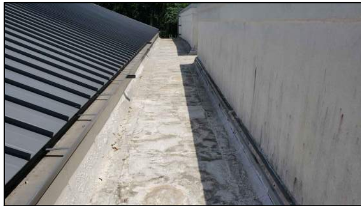
PHOTO # 11 ROOF AREA A1
