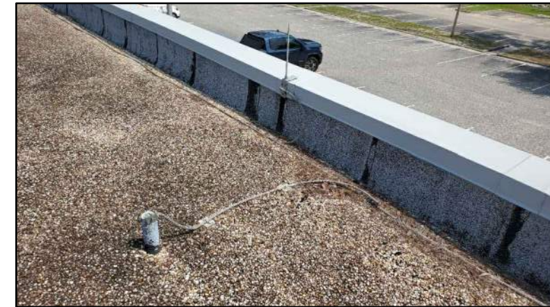
PHOTO # 6 ROOF AREA B
