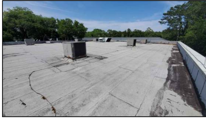
PHOTO # 2 ROOF AREA A
