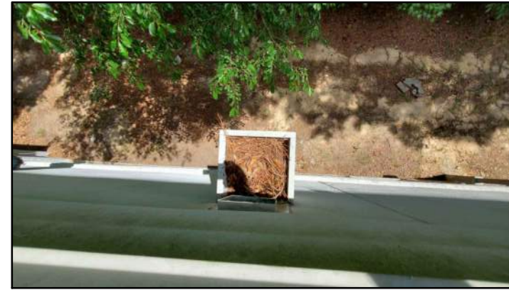
PHOTO # 6 ROOF AREA A
