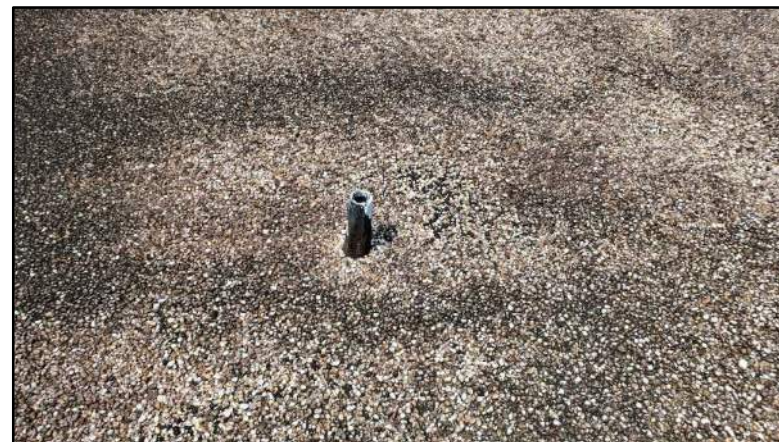
PHOTO # 8 ROOF AREA B
