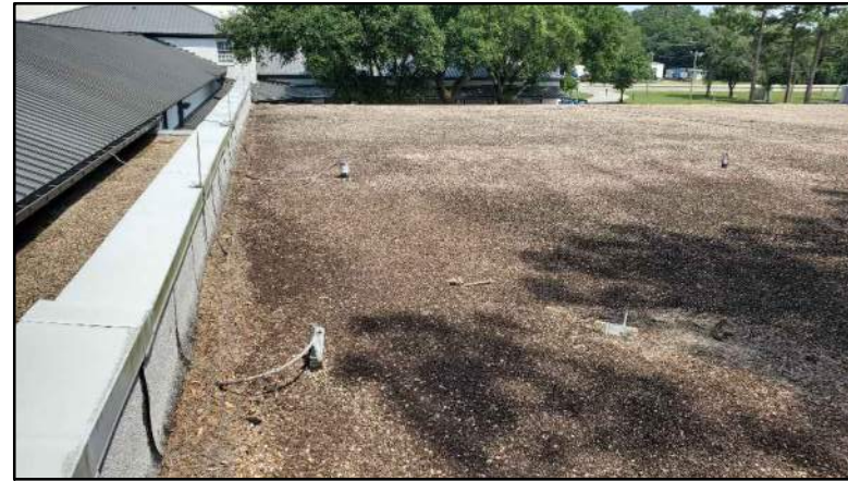
PHOTO # 2 ROOF AREA B
