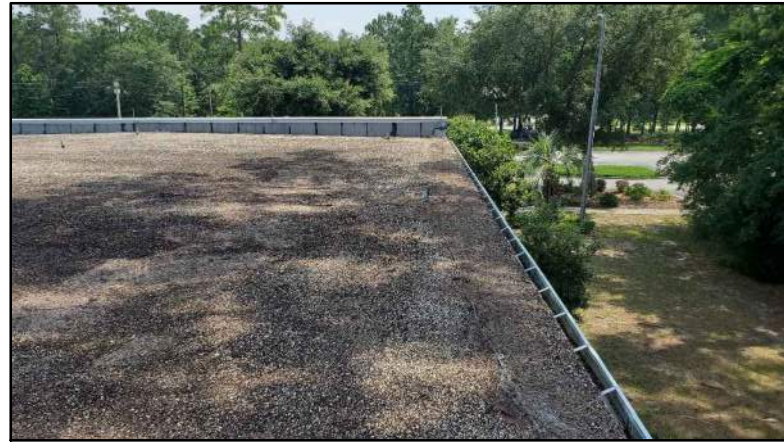
PHOTO # 1 ROOF AREA B
