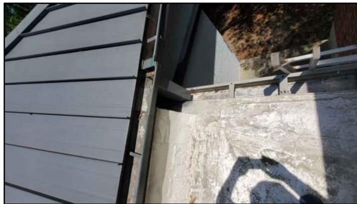
PHOTO # 8 ROOF AREA A1
