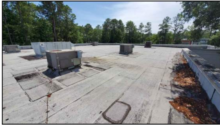
PHOTO # 4 ROOF AREA A
