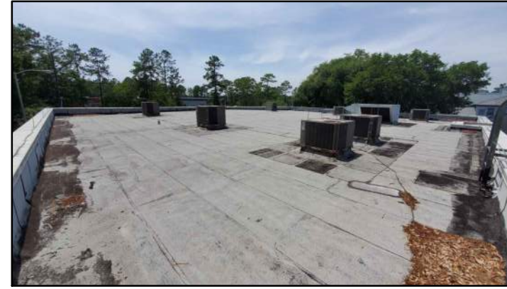
PHOTO # 3 ROOF AREA A
