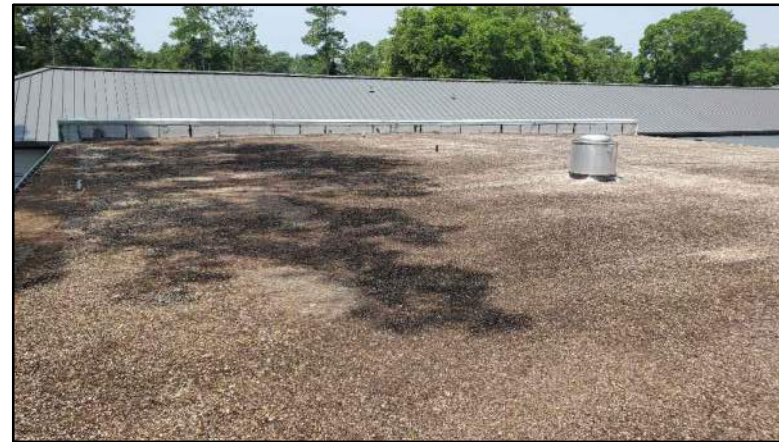
PHOTO # 5 ROOF AREA B
