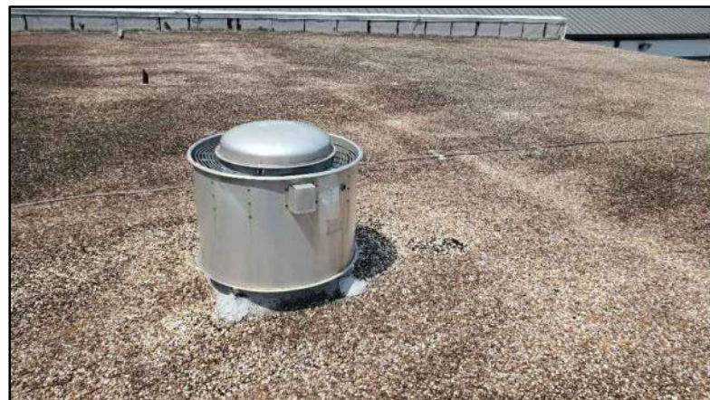
PHOTO # 7 ROOF AREA B
