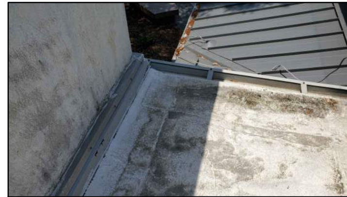
PHOTO # 12 ROOF AREA A1
