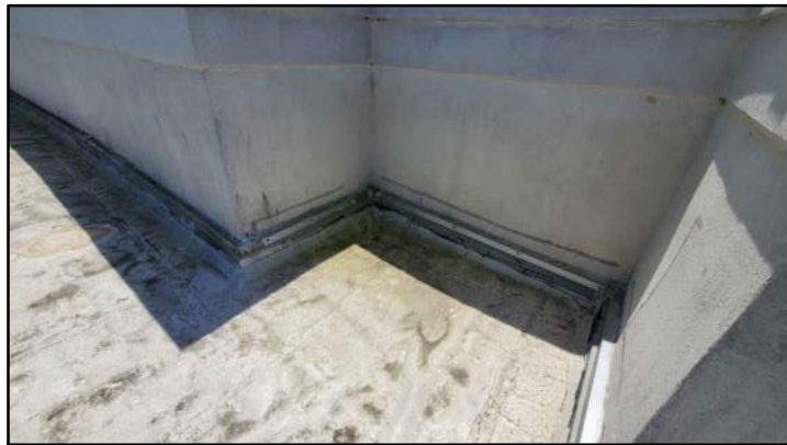
PHOTO # 10 ROOF AREA A1
