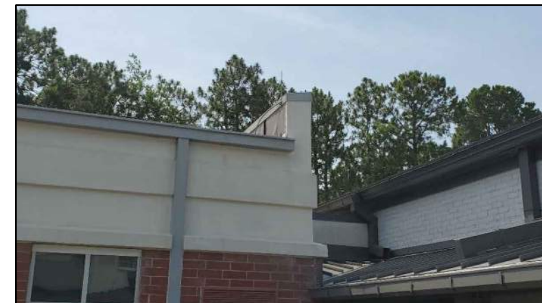
PHOTO # 9 ROOF AREA B
